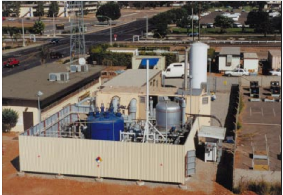
M-C Power's 250-kW MCFC demonstration unit at the Miramar Marine Corps Air Station, San Diego, California
