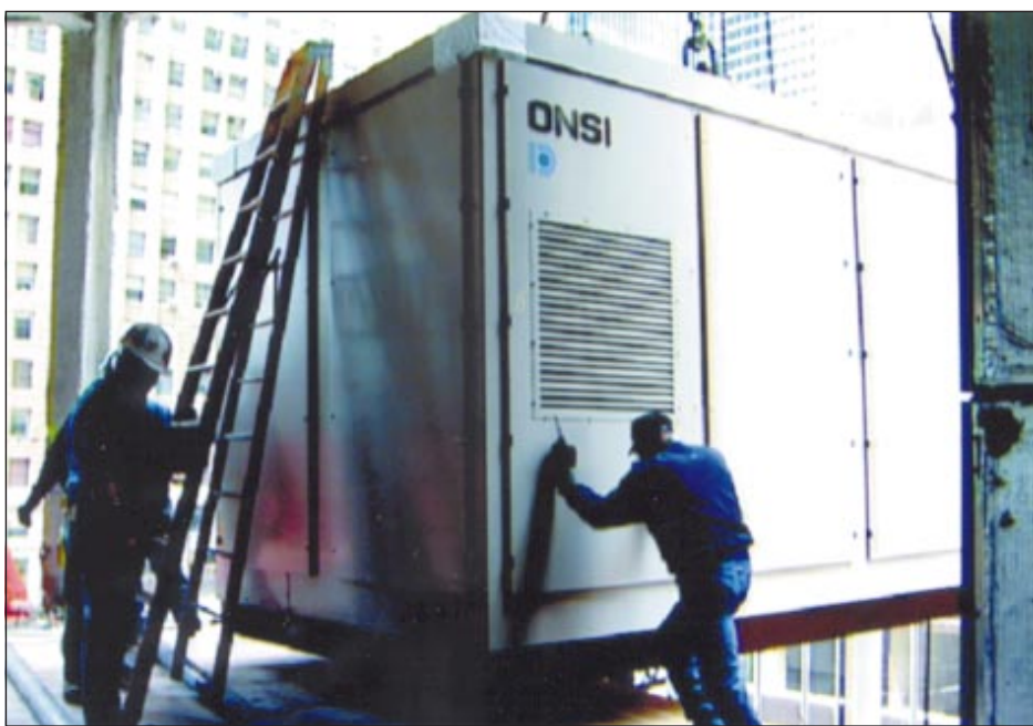
PAFC being installed at New York City's Times Square
